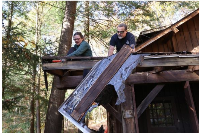
Emergency repair- Garfield front porch roof
