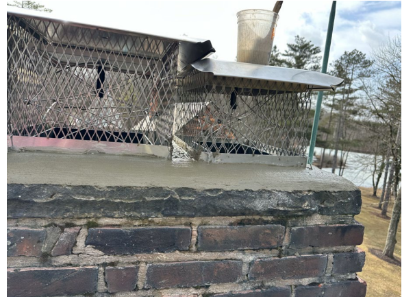
New chimney cap and screen to exterior fireplace and new chimney cap, screen, and spring-loaded damper to living room and basement.
