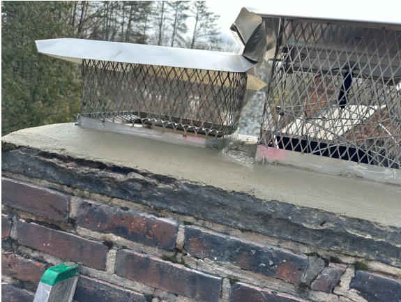
New chimney cap and screen to exterior fireplace and new chimney cap, screen, and spring-loaded damper to living room and basement.
